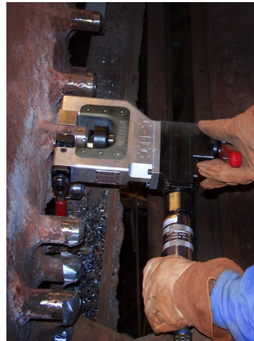
The C-HOG is ideally suited for beveling small bore heavy wall tubes with a high percentage of chrome, stainless steel and other hard alloys.
